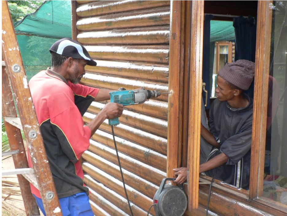
Tshabu on the left, busy repairing a log house.
